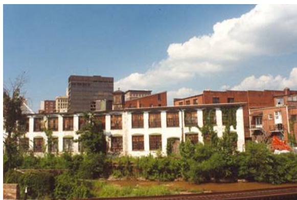
Figure 14: Old Wyche Pavilion, pre-renovation (Source: City of Greenville)
