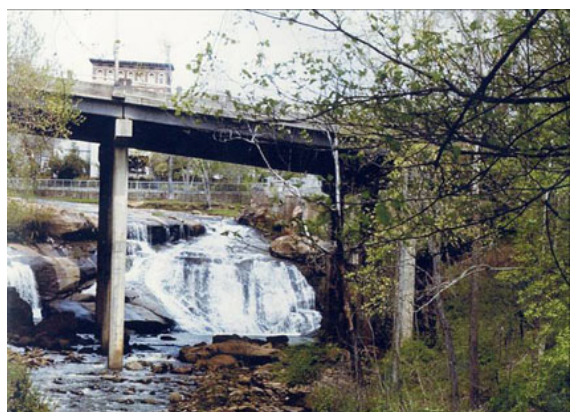
Figure 16: The demolished Camperdown vehicular bridge. (Source: City of Greenville)
