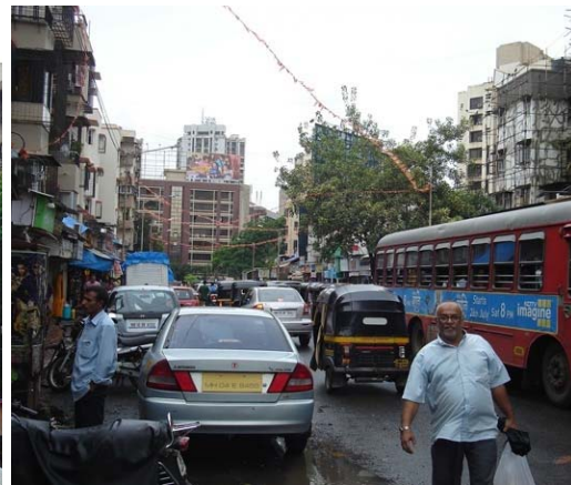
Fig. 7: Poorly maintained buildings
