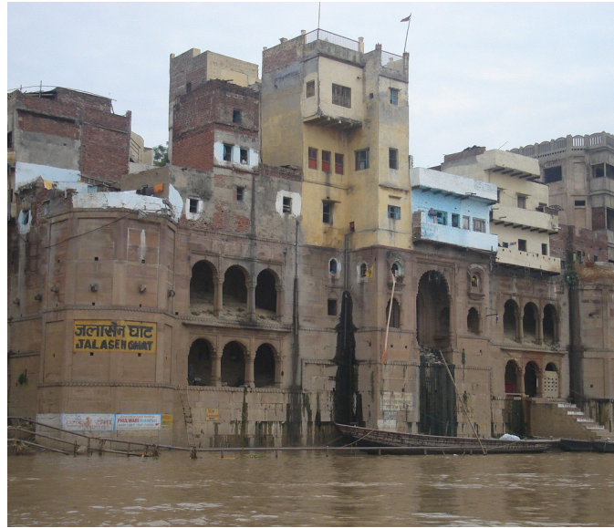
Figure 3: Recent construction incompatible with existing historic fabric in form, materials and methods.
