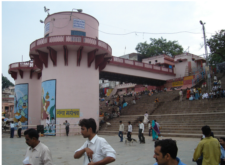
Figure 7: Sewage treatment towers at Dashashwamedha Ghat. While fulfilling a vital need, their form and placement compromises the integrity of the sacred space.
